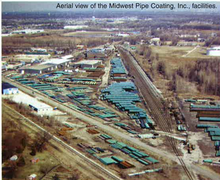
Aerial view of the Midwest Pipe Coating, Inc., facilities.
